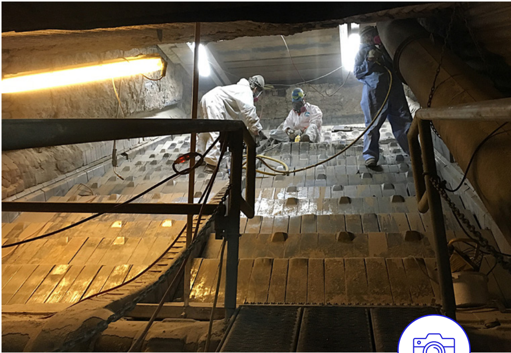
Critical outage service-stoker grate
